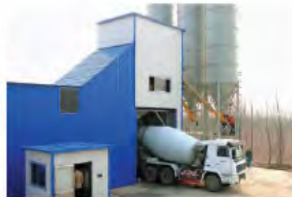
Heat Preservation Concrete Mixing Plant
