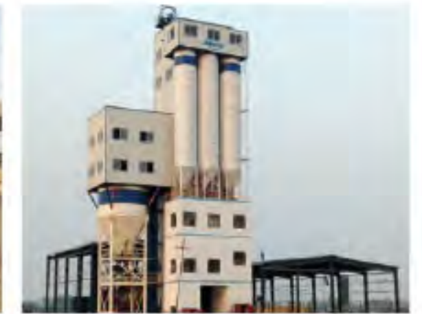
Dry Mortar Mixing Plant
